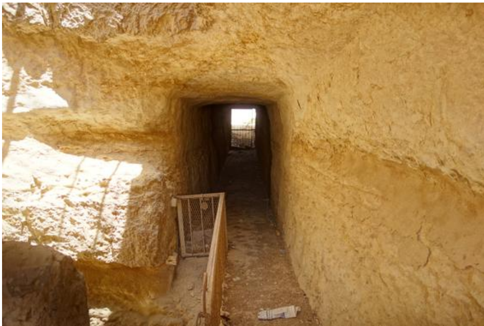
Analysis of the interior of the tunnel itself seems to confirm this function as a rainwater outlet to the south. A vertical shaft was dug in the roadway itself, in the southern sidewalk, but this appears to have been dug at a later date.
